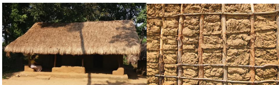
Figure 10, 11. Typical mud hut in Sri Lanka and wattle and daub technique
