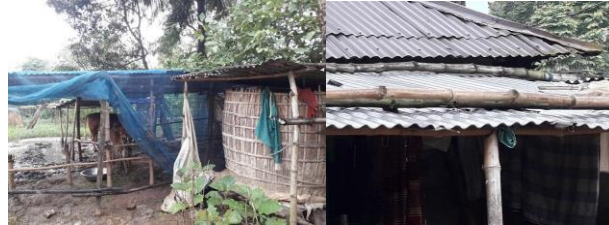
Figure 5, 6. Cattle and hen shade, Roof with CI (Corrugated Iron) sheet, supported by bamboo.
